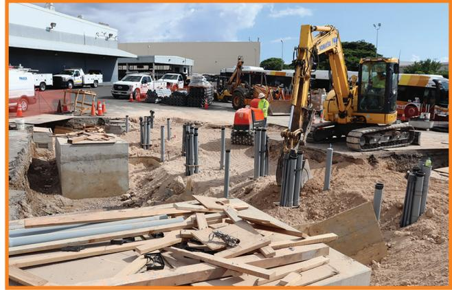
Photos above: Construction crews working on the new charging stations for the new electric buses.
